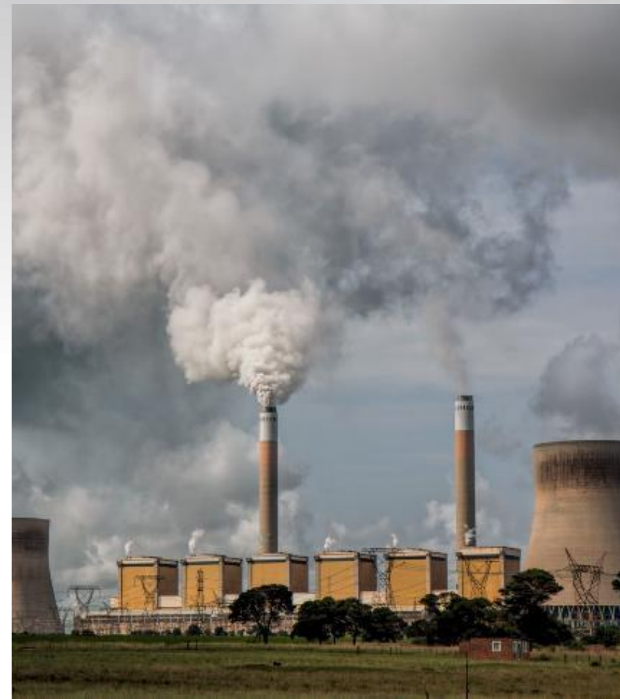
Greenhouse gases emission monitoring
